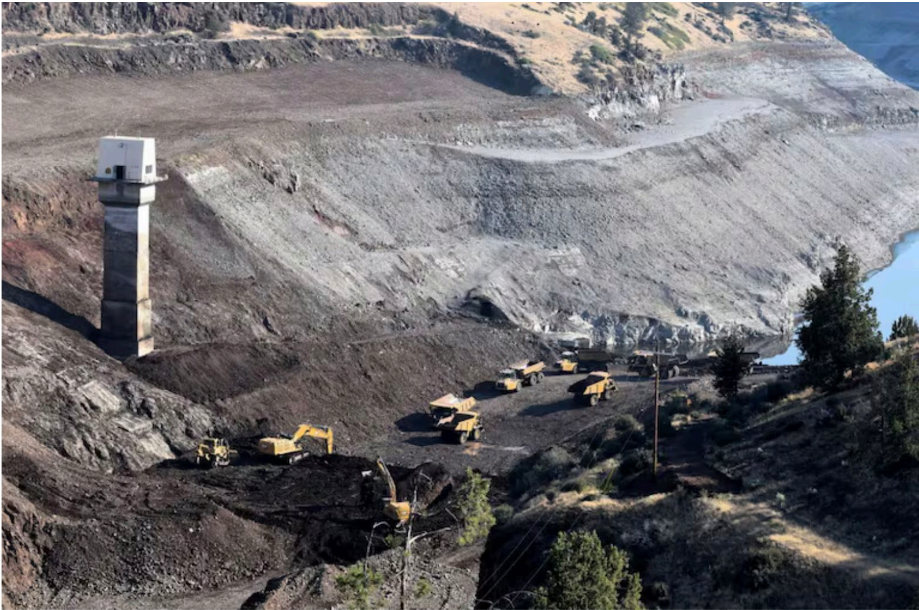
Scoop by scoop, crews from construction company Kiewit are deconstructing the massive earthen barrier that was Iron Gate dam, July 26, 2024.
