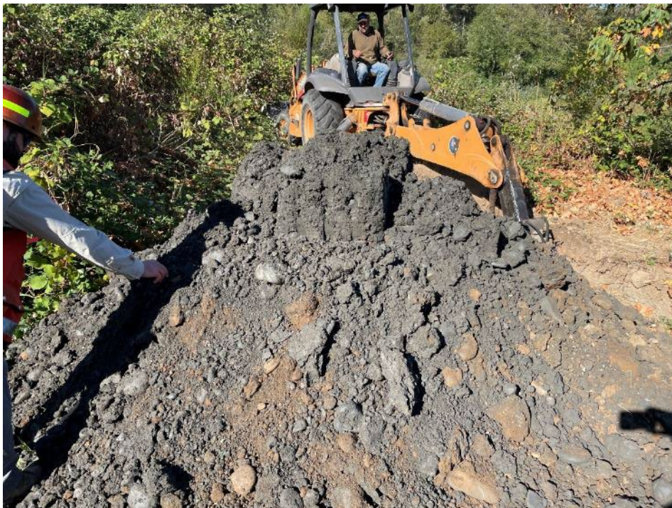
Top left – disturbed fill layers in top 4 feet. Top right – Material below 5.5 feet depth comprised of sandy silt with gravels. Bottom – spoils pile mostly showing deeper sandy silt and clay loam layer, some gravels and cobbles up to 6 inches diameter.
