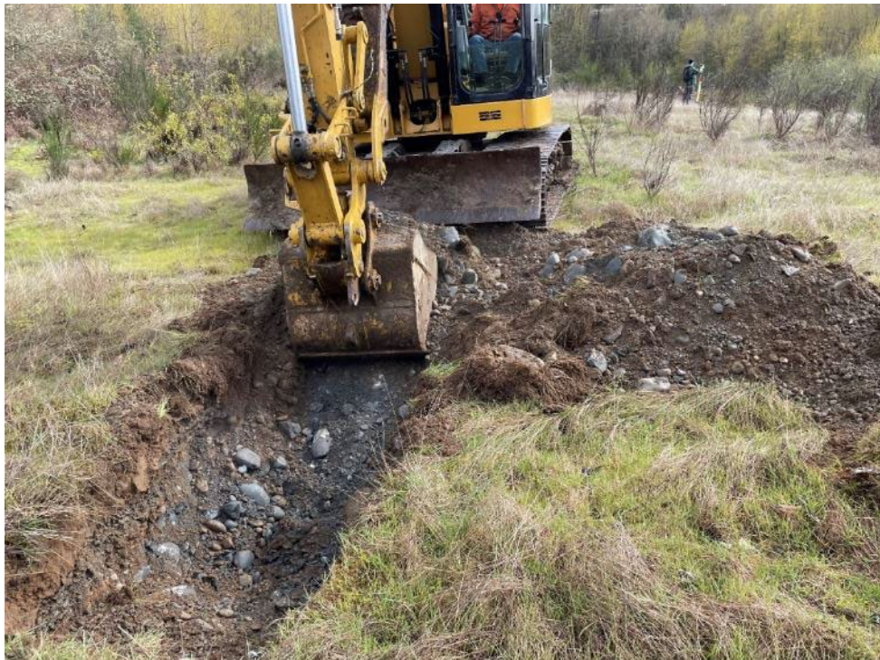
Top – Consolidated clay and sand layers mixed with cobbles.
