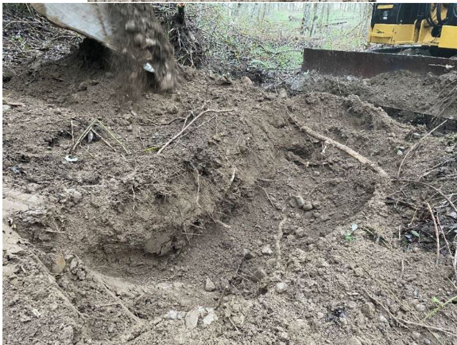
Top & bottom – Gravel and cobbles in fine matrix
