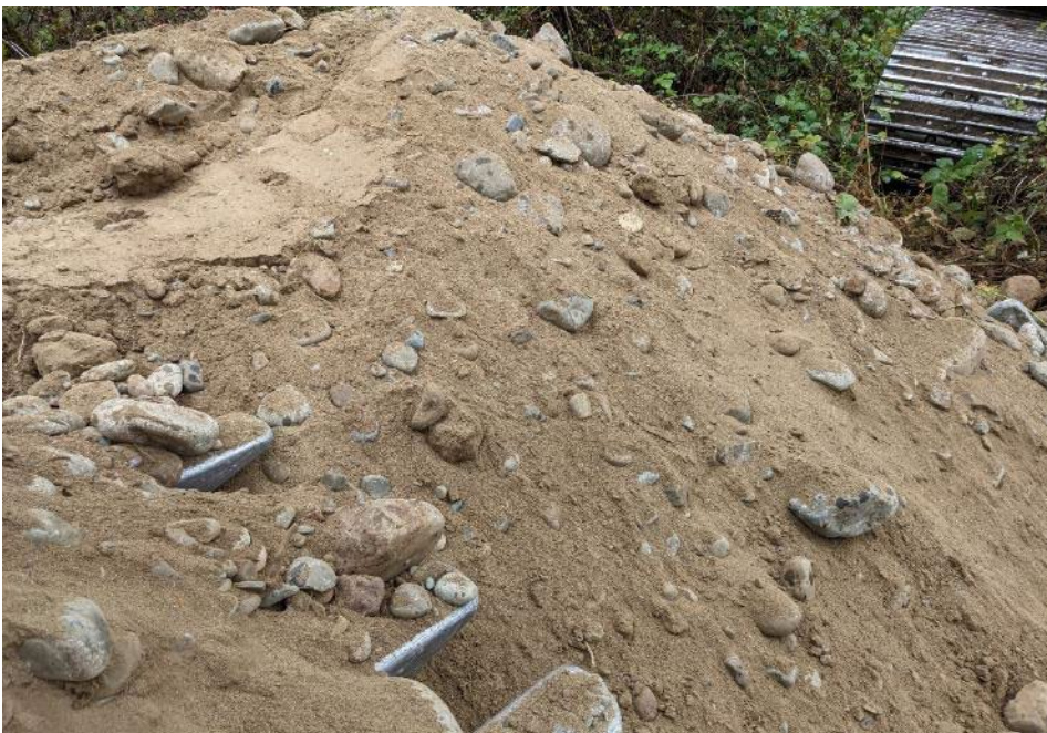
Top - Pit in berm, sandy loam with cobbles at 7 feet; Bottom - close up of spils pile from bottom of pit
