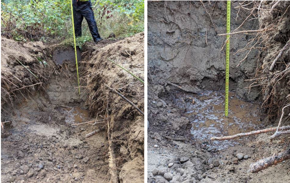
Left - Pit with thick roots at top, silty sand; Right - Close up of groundwater at approximately 6 feet, pit caving in at 6 feet
